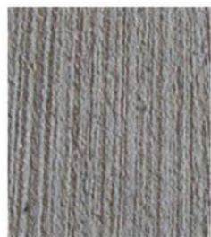
Unsealed Brushed Concrete
