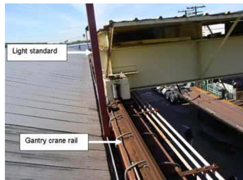
The rail on which the gantry crane rides and its close proximity to the light standard.
