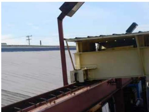
Gantry crane and light standard against which the victim was crushed.
