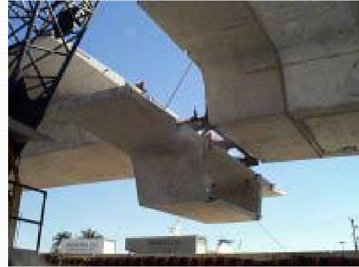
Concrete Segmented Bridge
