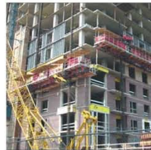
Preventing falls and fatalities with tie-in scaffolding (5)
