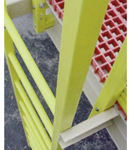
A high-exposure area for an accident to occur is getting off an elevated platform to the fixed ladder.
