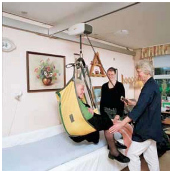
Photo 1. A room-traversing ceiling lift in operation.
