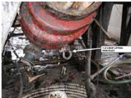
Lifting shackle of blowout preventer (BOP).
