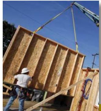
From top: Photo 1 shows an example of on-site built modularization while Photo 2 shows workers hoisting a prefabricated module.
